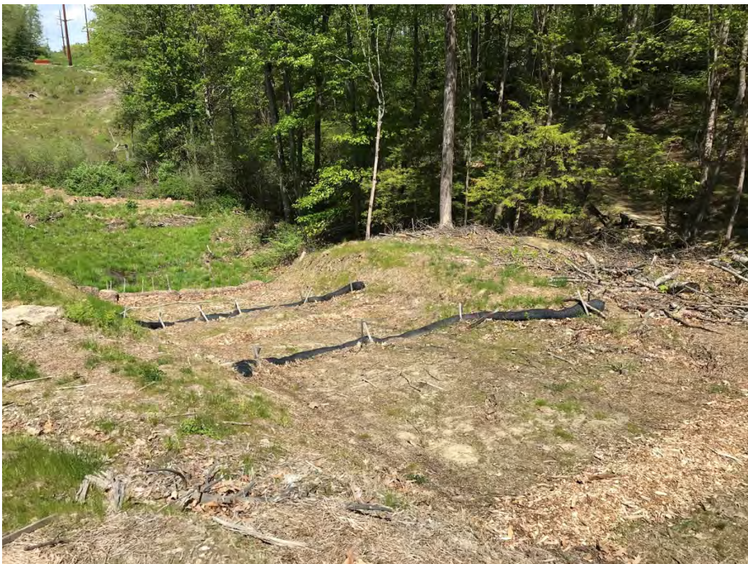
Fig 8: Lower portion of slope between Strs. 28 and 29. Viewing northeast. (05-17-21)
