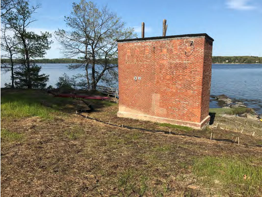
Fig 1: Slope leading down to cable house and salt marsh restoration at the west side of the bay. Viewing northeast. (05-17-21)
